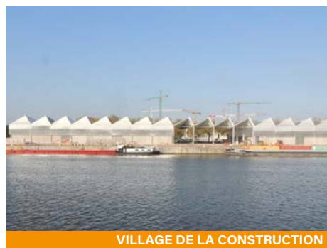
VILLAGE DE LA CONSTRUCTION
