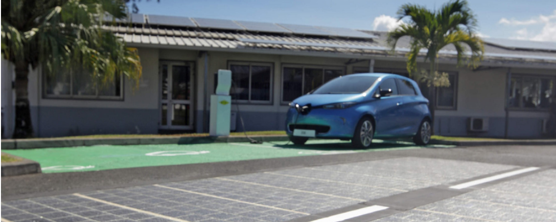
Example of implementation the “Wattway” in the city of Le Port (La Réunion, France) © Colas group
