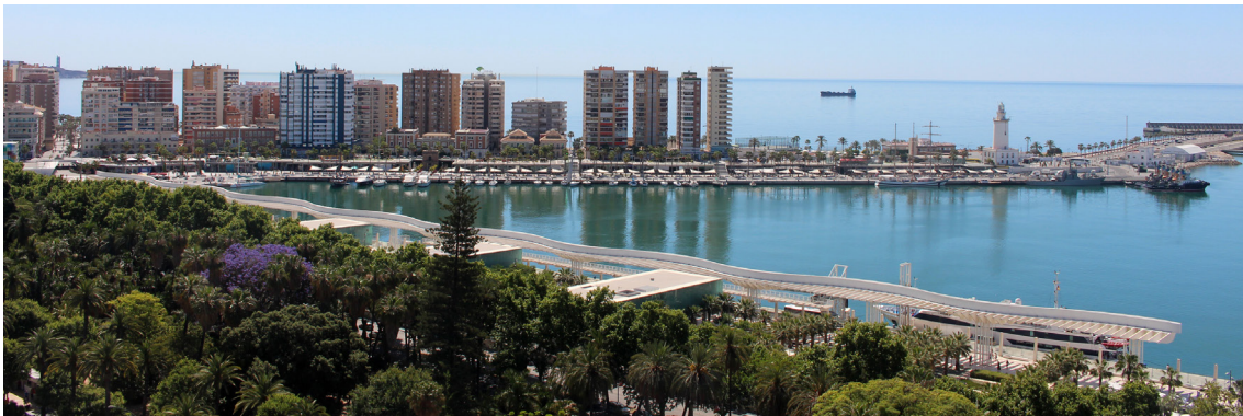
Docks 1 and 2 of the port of Malaga ©Malaga port
