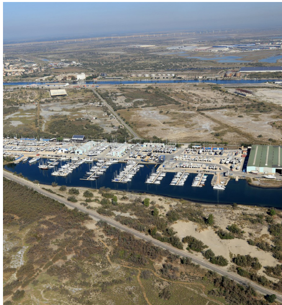
Aerial perspective of Port Napoléon, the private yachting area managed by Port Adhoc in Port-Saint-Louis-du-Rhône
