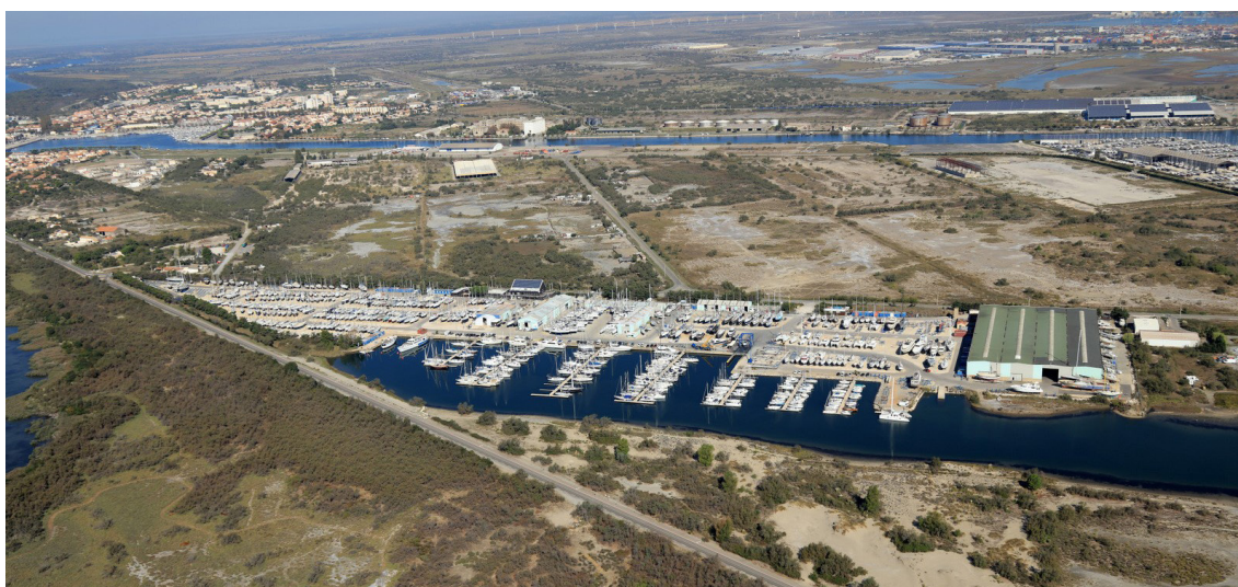
Aerial perspective of Port Napoléon, the private yachting area managed by Port Adhoc in Port-Saint-Louis-du-Rhône
