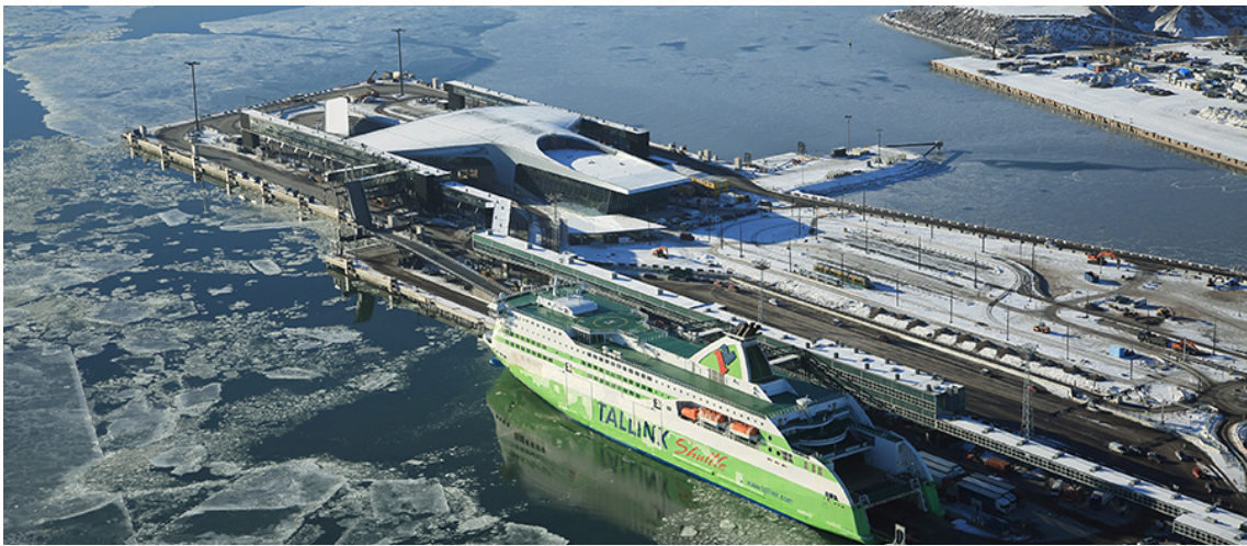
West Harbour T2 ©Port of Helsinki
