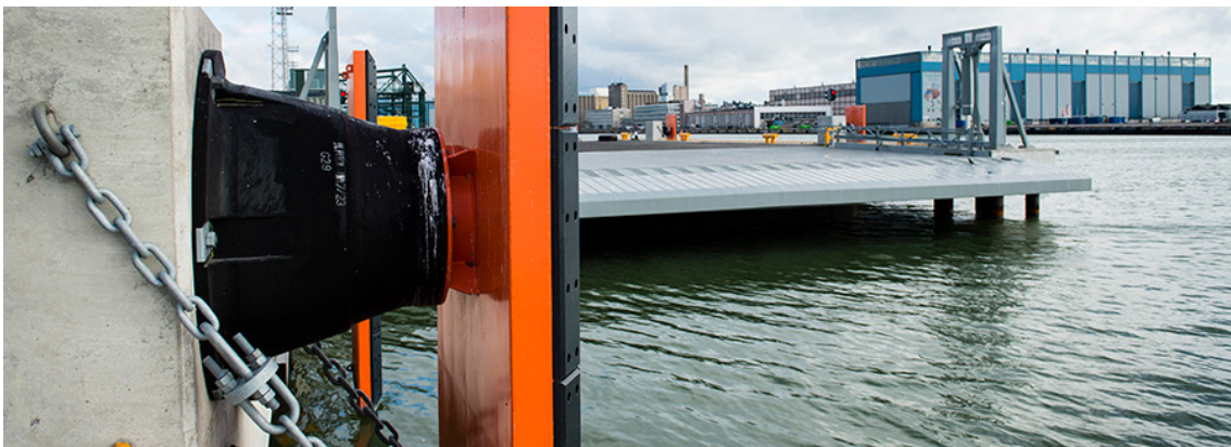
West Harbour Automooring ©Port of Helsinki
