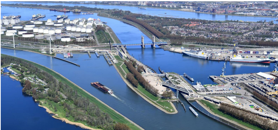
Aerial photo Theemwegtracé, Botlek. Danny Cornelissen. Provided by the Port of Rotterdam.
