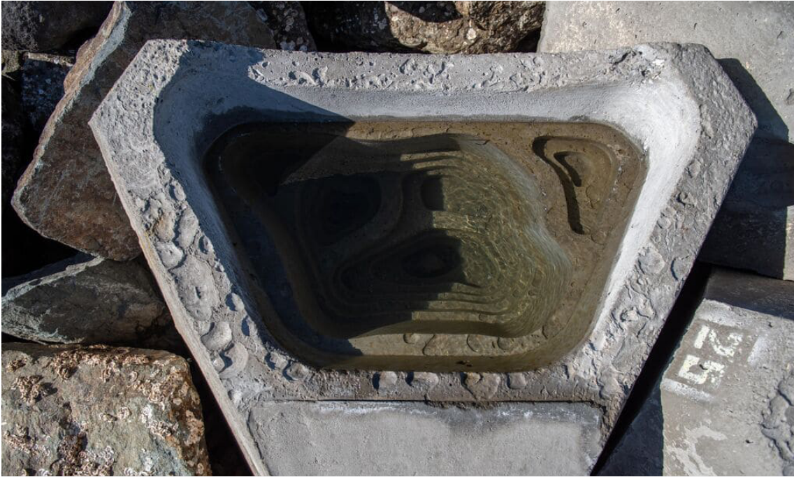
ECONcrete Tide Pool. (©Port of San Diego)
