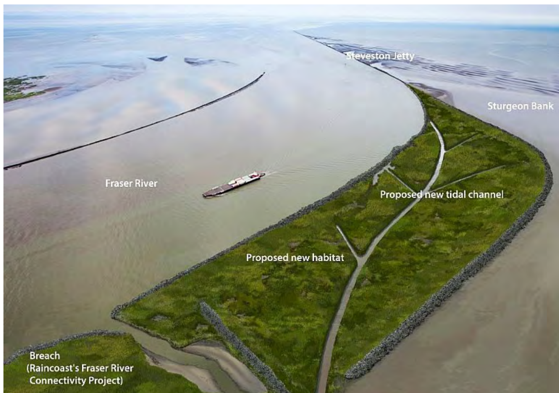
South Arm Jetty Tidal Marsh @ Puerto de Vancouver
