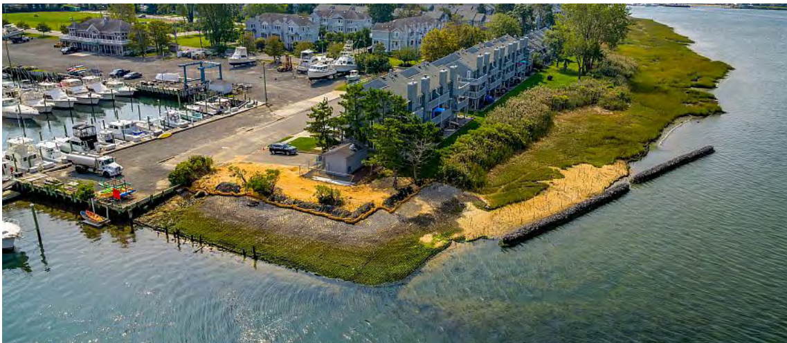
Neptune project – Shark River Island, Neptune, New Jersey – After © ECOconcrete
