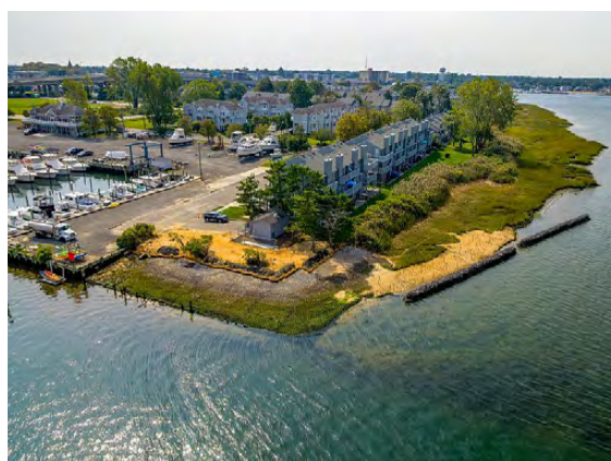
Neptune project – Shark River Island, Neptune, New Jersey – After © ECOconcrete
