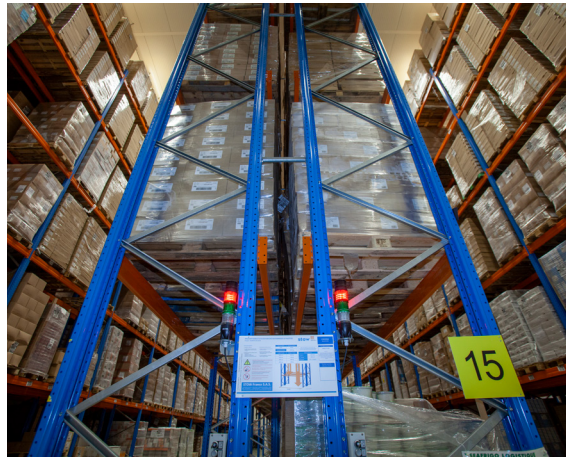
Interior of warehouses © Seafrigo
