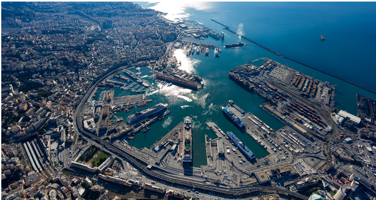
Aerial view – Port of Genoa. Source: Western Ligurian Sea Port Authority
