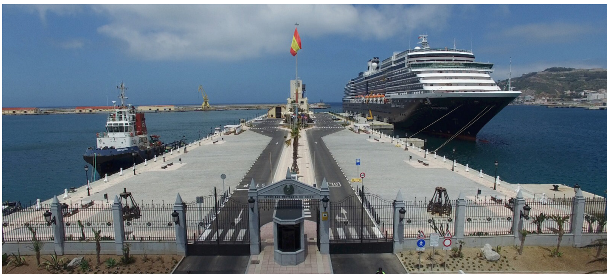
Cruise pier of the Port of Ceuta. Source: Port of Ceuta
