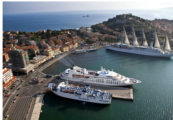
Portoferraio cruise port. Source: North Tyrrhenian Port Network Authority
